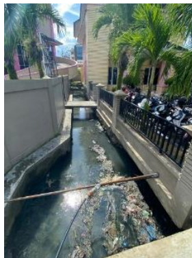
Pict 1. Primary Drainage Channel at Faculty of Economics
