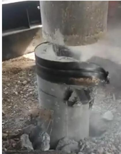
Gambar 10. Cutting Pile
