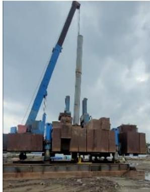
Gambar 5. Clamping Pile
