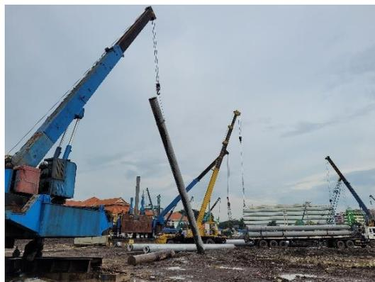
Gambar 4. Lifting Pile
